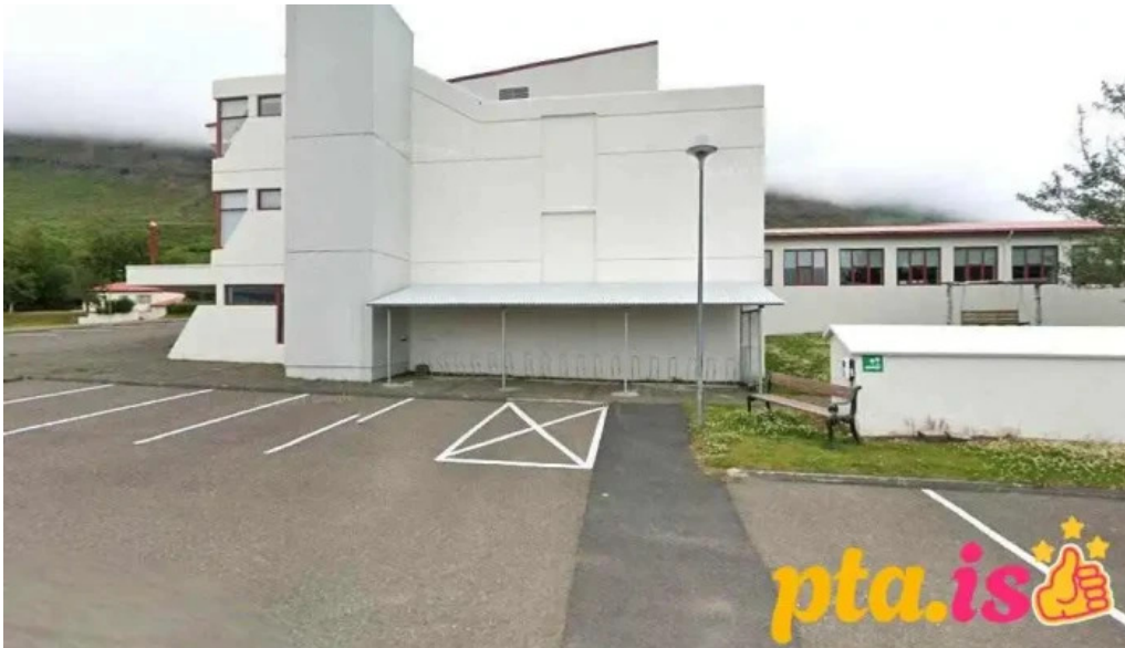
Isorka charging station neskaupstaður
