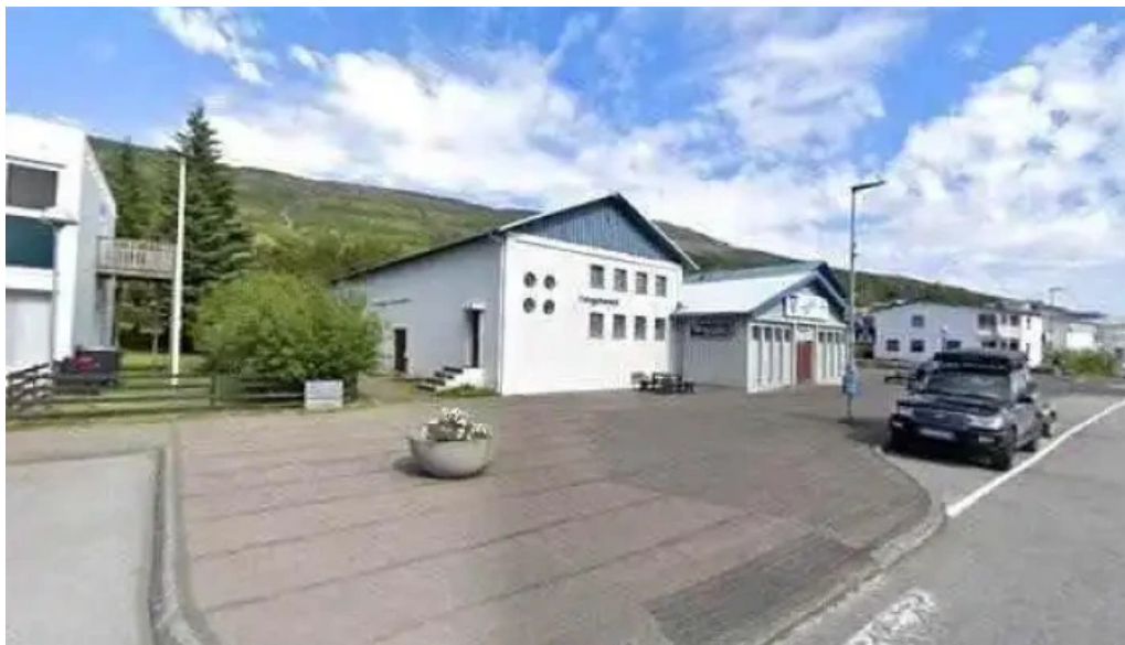
Posthus eskifjordur street view 360deg
