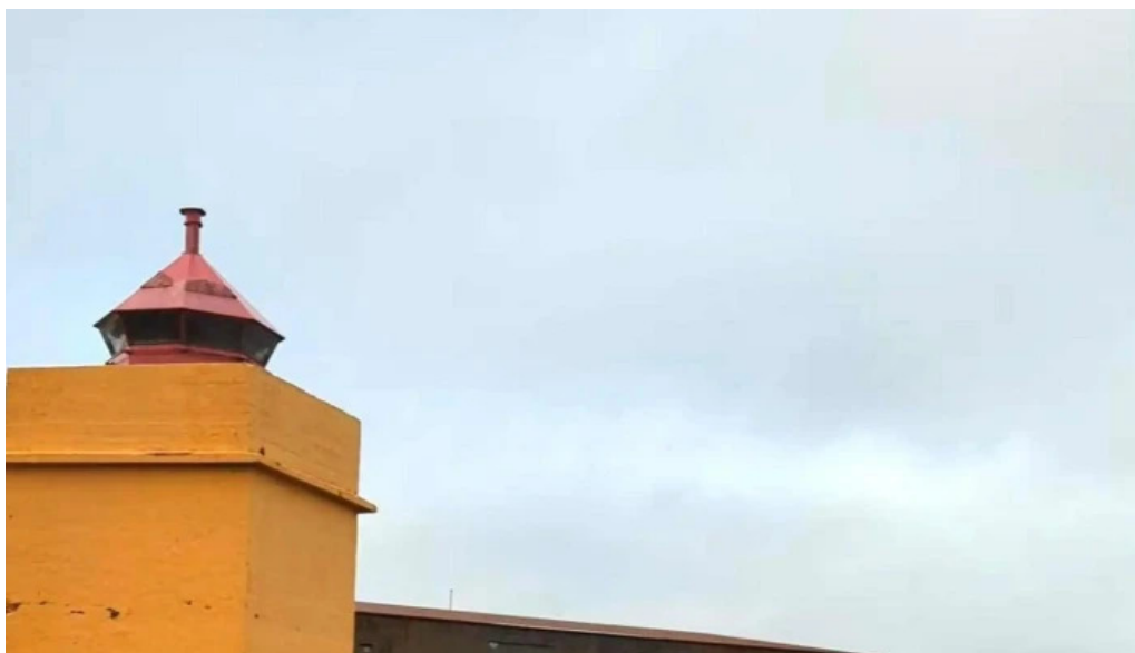
Vatnsnes lighthouse athugasemdir
